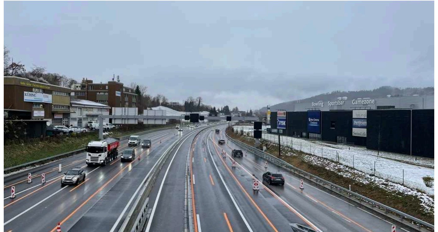
Berne Agglomeration: Extension of road infrastructure for “bottle neck” elimination for traffic during peak hours
